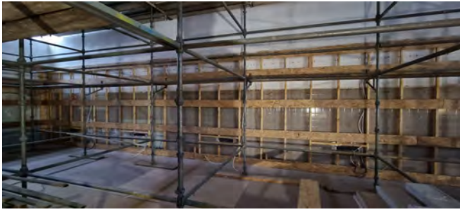
TIMBER FRAMEWORK BEFORE INSTALLATION OF IMPACT PANELS
